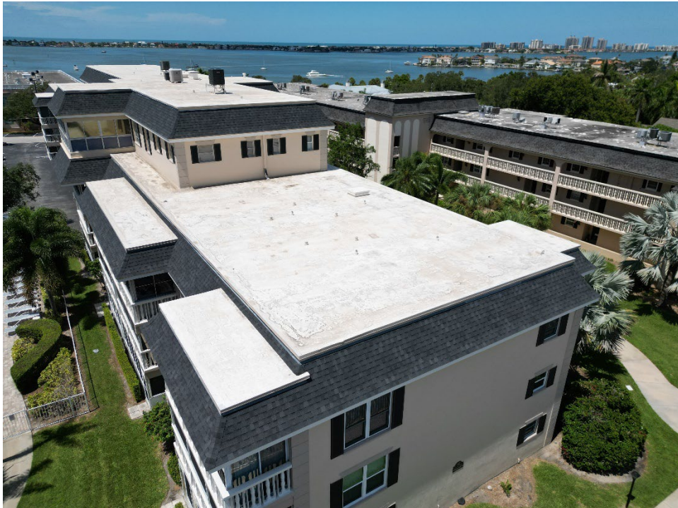
2. View of the main roofs.
