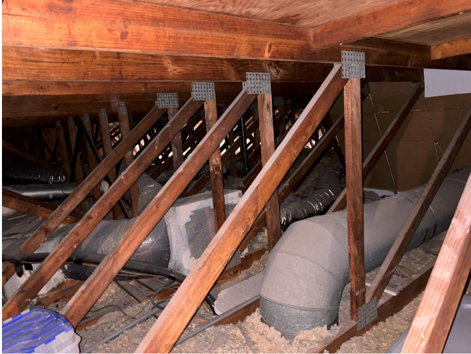
3. View of typical roof framing.
