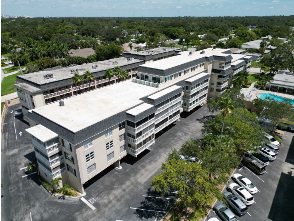
1. View of the subject building.
