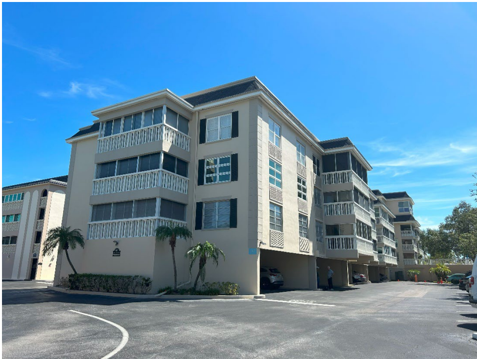
12. View of the west elevation of the building.
